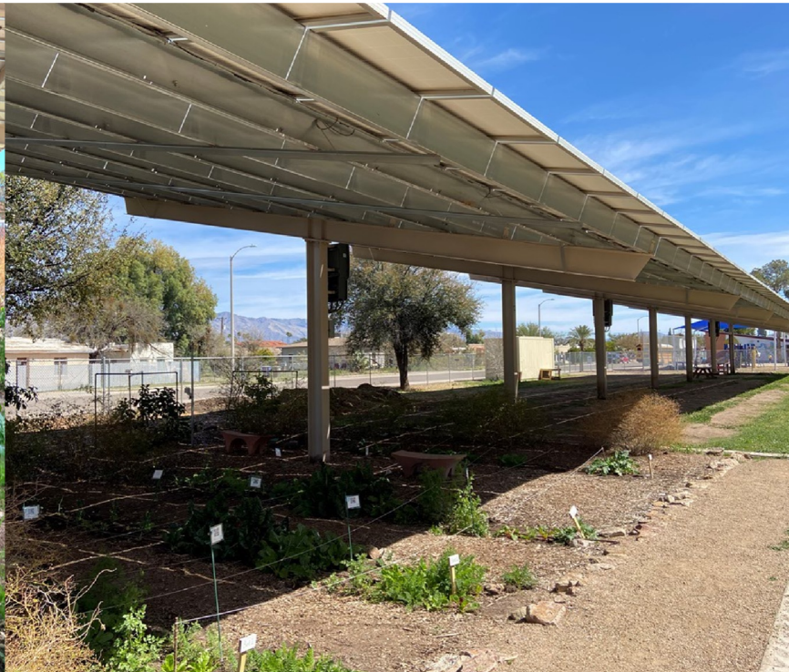
Solar Garden at Manzo Elementary
